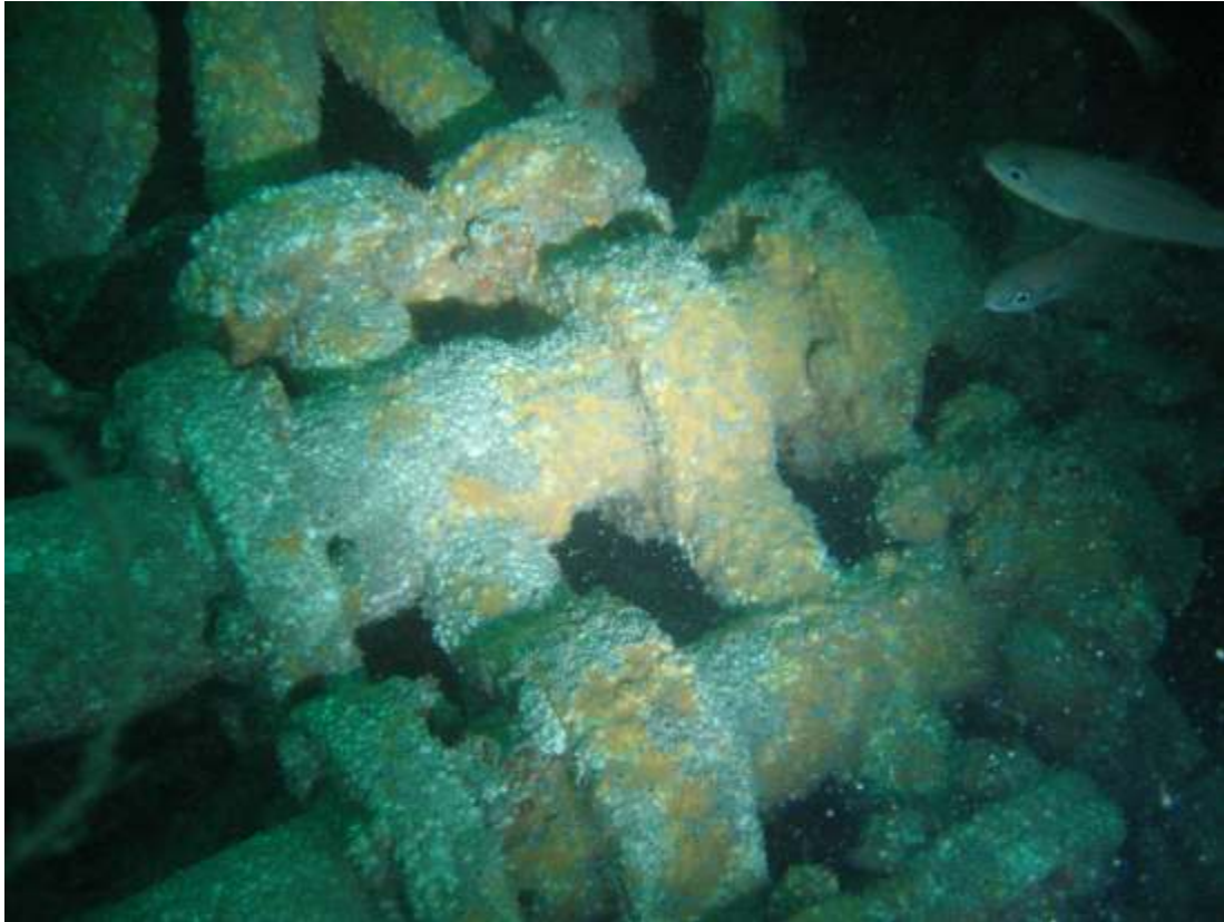
Plate 8. Flanged and bracketed pipes, possibly associated with the boilers or engine room (Courtesy of Keith Rimes)
